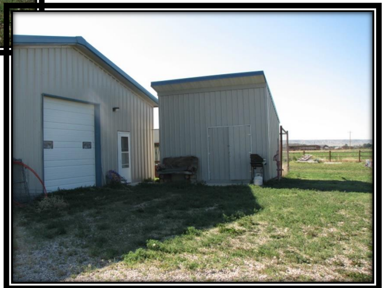
Storage Shed with Electricity
